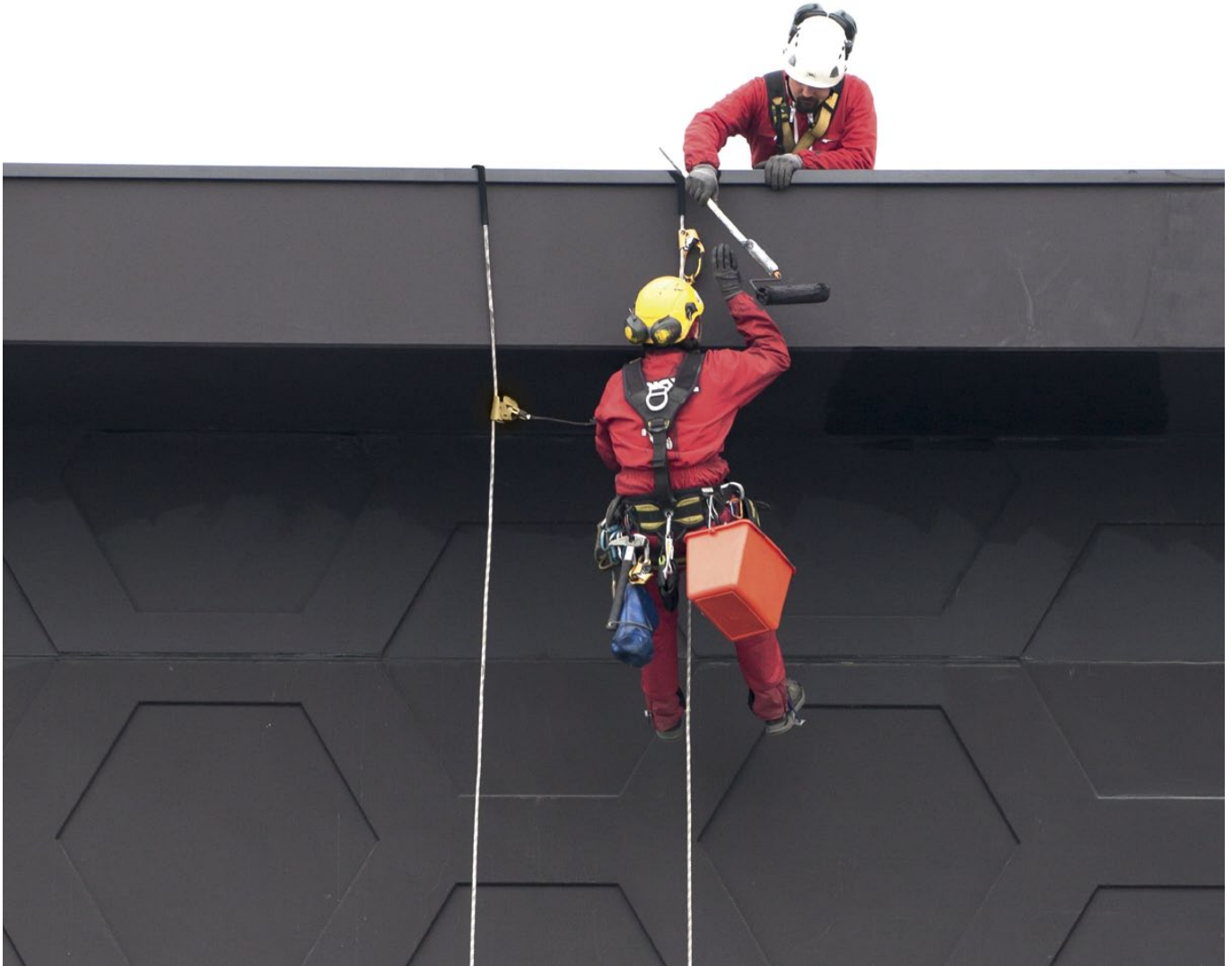
Prisme, Petzl Batiment M3, Crolles, Isère, France © Lafouche
