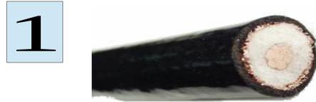
Cut off cable tail right-angled with a small metal saw. The inner conductor has to be kept absolutely round.
