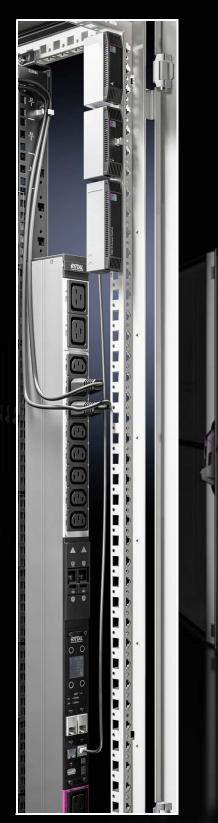
Application-specific sensors may be incorporated into the central monitoring system directly via the PDU's CAN bus interface.
